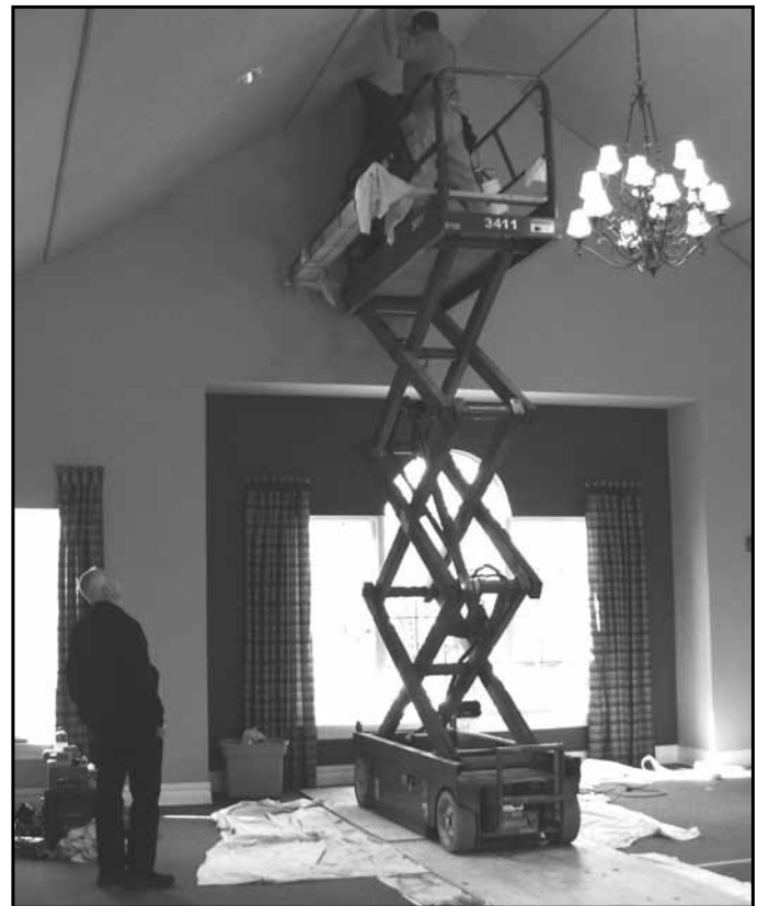
Mike Segal checks on the progress of the acoustical ceiling
