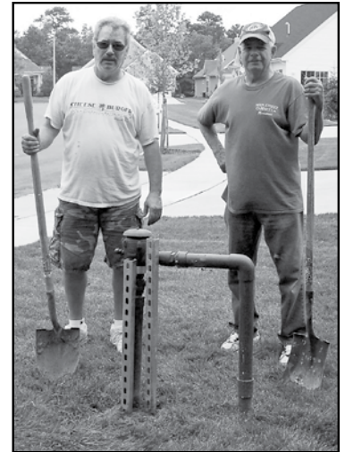
Joe Carluccio & Bill Hofmann installed security on backflow preventer.
