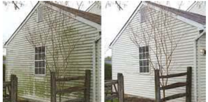
Mold on house exterior on left and after power washing on the right
